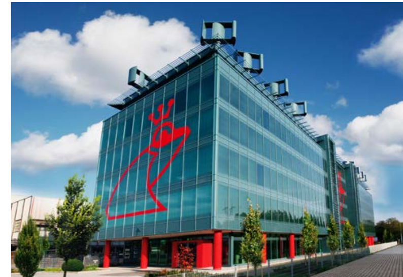
The new administration building of the Mainz-based family company Werner & Mertz (famous for the Frosch and Erdal brands). Special feature: Thanks to photovoltaics, the building produces more energy than it uses.
