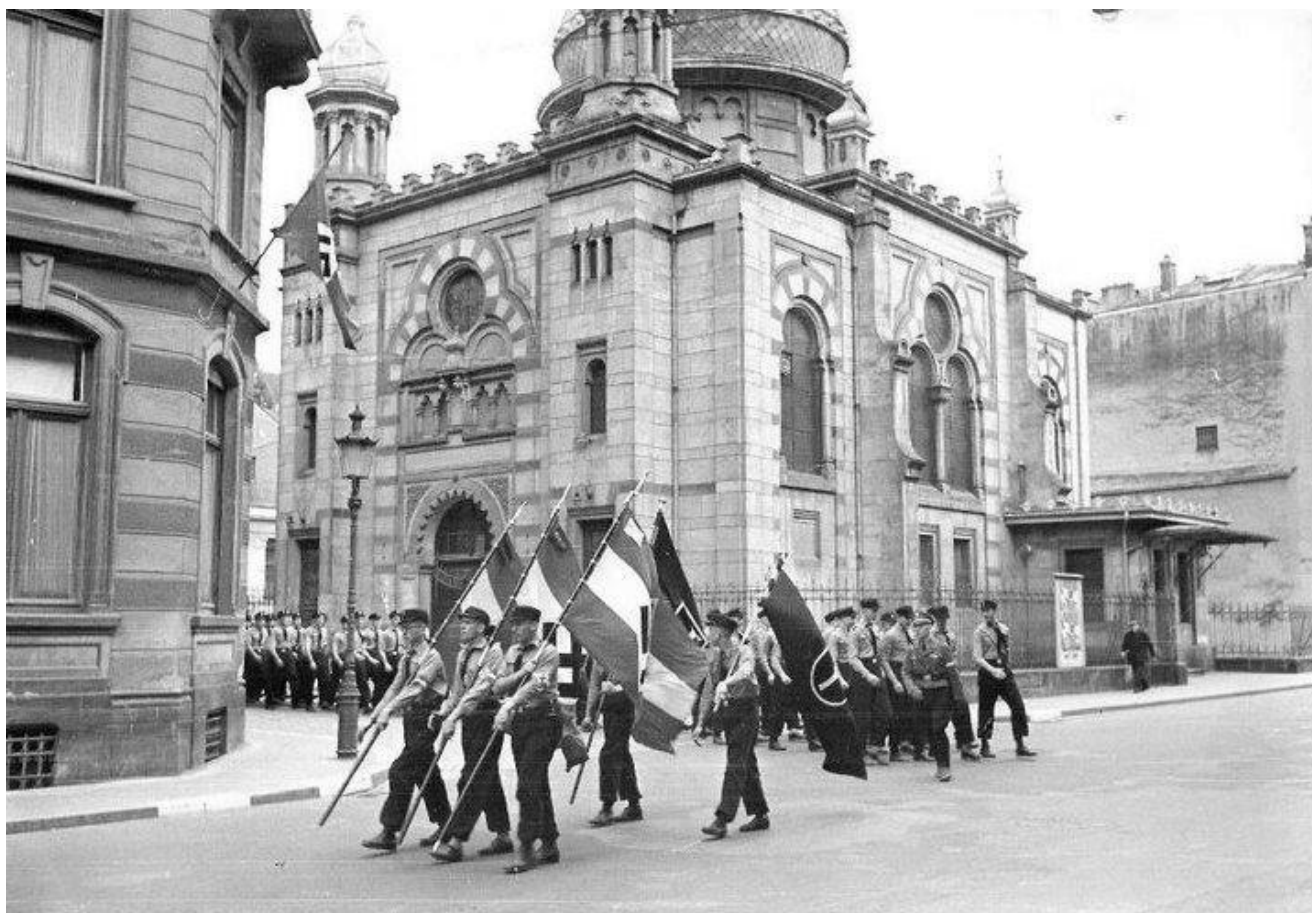
A 1941 Nazi parade in front of the Luxembourg City synagogue, which used to be at the corner of Rue
