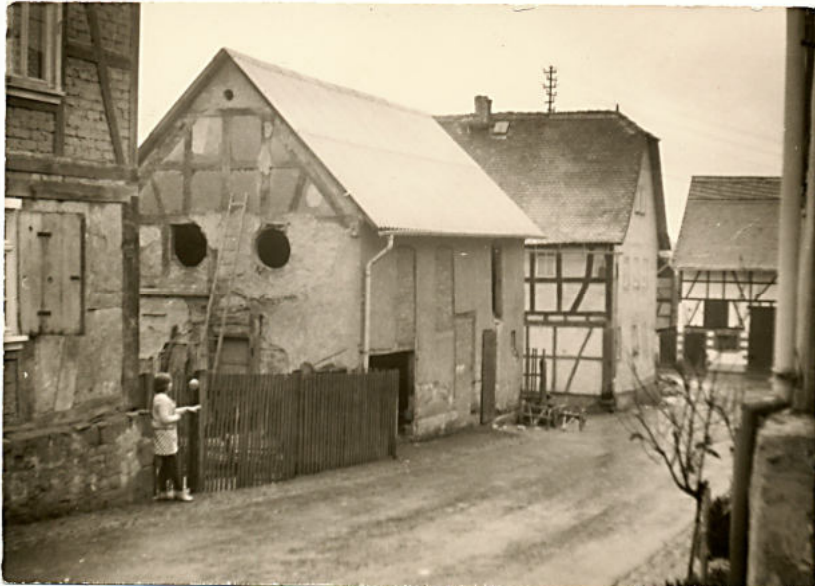
Einartshausen Synagogue, 1960s prior to demolition in 1964, with thanks to Dr Brumhard
